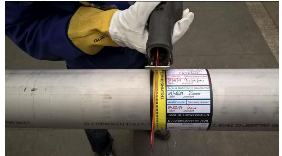
Clearly identified and marked pipeline
